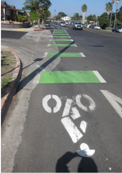
Clairemont Drive Class II Bike Lane with buffer zone and conflict striping across the intersection.
